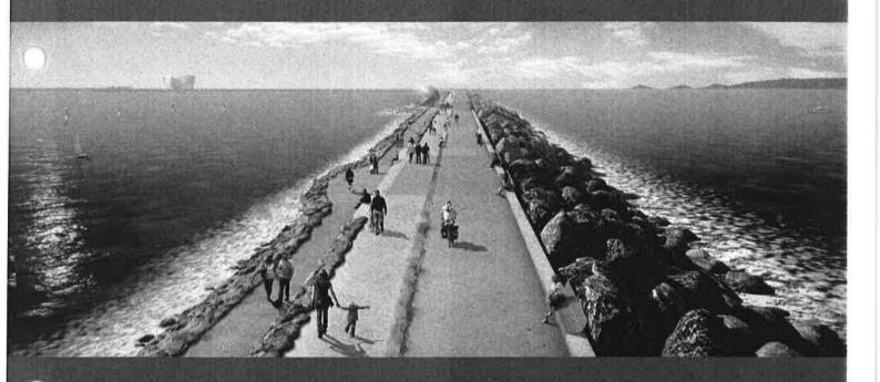
Tidal lagoons are seawall structures that impound areas of water. As the tide rises and falls, water is held back and its energy is harnessed as it passes through turbines set within the seawall.
